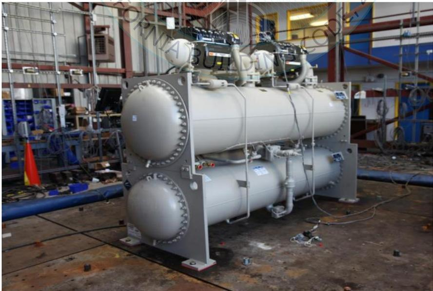
UUT3 was base mounted - rigid to the table using eight (8) 1" SAE Grade 8 bolts, washers and a 1/4" ribbed neoprene pad under each mounting foot (4).
