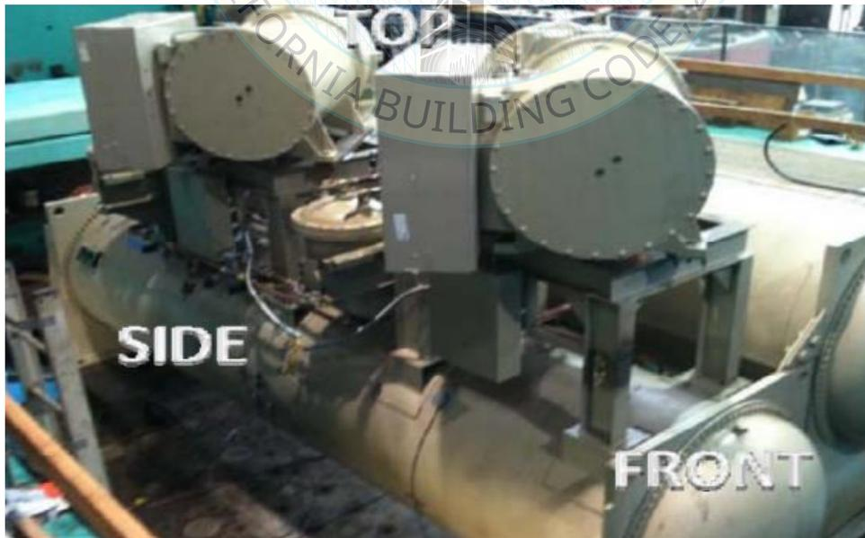
UUT2 was base mounted - isolated on 1/4" neoprene pads with eight (8) 1" Grade 8 bolts.
