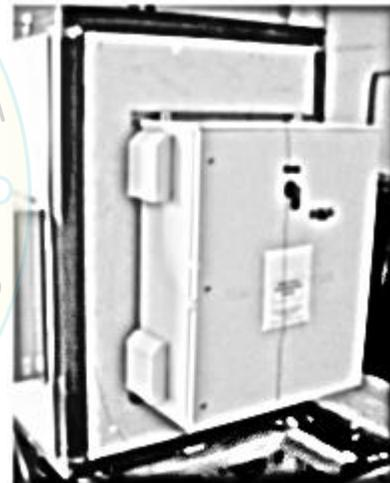
**UUT-7: 40HP 460V Drives in NEMA 3R Enclosure on Unistrut Backing**
