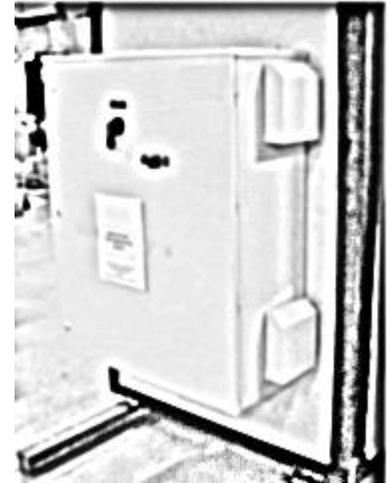
**UUT-6: 75HP 460V Drives in NEMA 3R Enclosure on Unistrut Backing**
