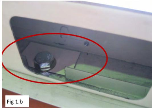
1. Figures 1.a and 1.b show the stiffener plates added to the base channel at each mounting bolt location. Each stiffener plate was 4"x2.25" with a .875" diameter hole. Each plate was made of pre-painted G60, 10 gauge steel with a nominal thickness of 0.138".
